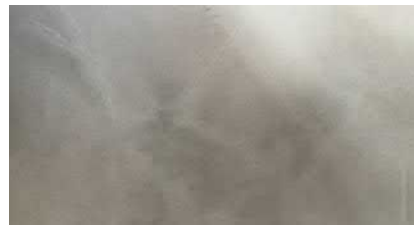
Trowelled micro cement smoothed MineralSphere®
