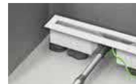
Plumb in drain
